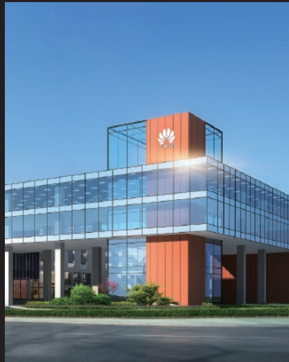
Huawei Cloud Computing Center
