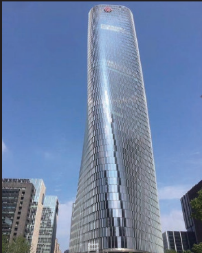
Bank of China Data Center
