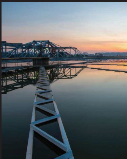
ABU DHABI Water Supply Project
