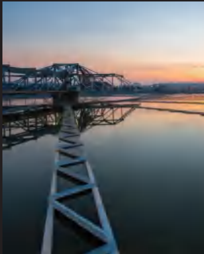
ABU DHABI Water Supply Project
