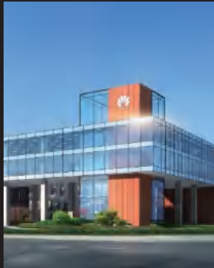
Huawei Cloud Computing Center
