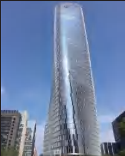
Bank of China Data Center
